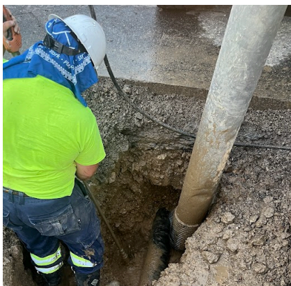
Recent water department projects including repairing a water main break at Xenia Ave. and Corry St.
